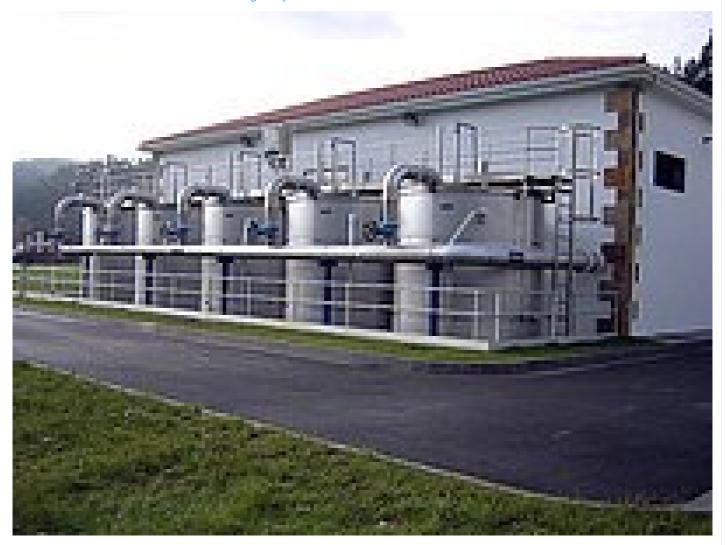
Filtration of biologically treated wastewater serves for removal of suspended solids (suspensa) remaining in clarifier effluents. Such suspensa contain about 50 % carbon, almost 10 % nitrogen and over 1 % phosphorus.
