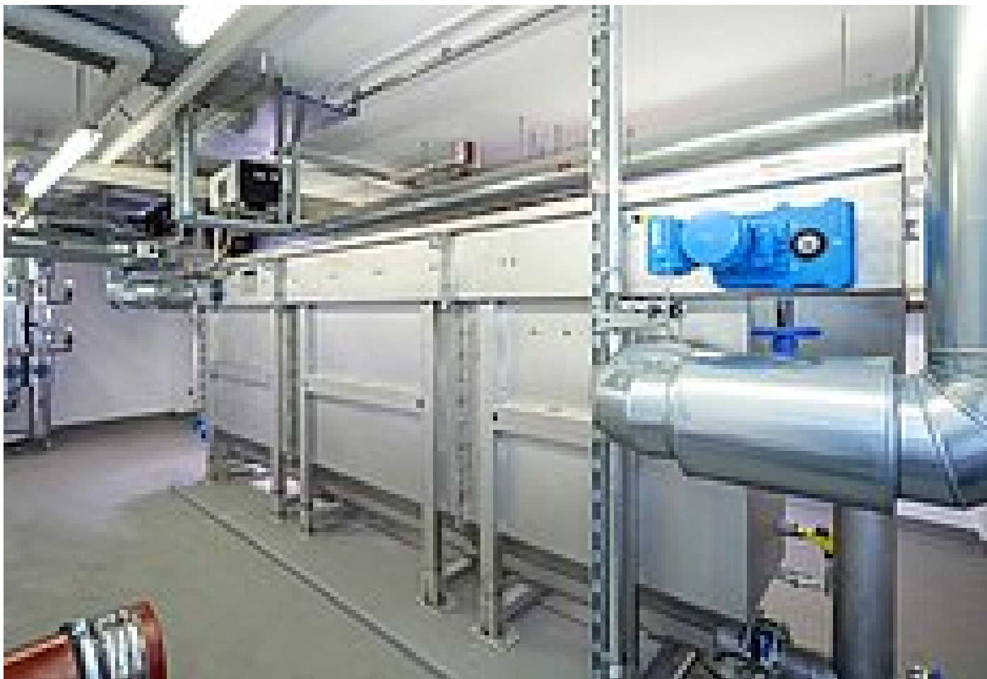
Flanged version of a HUBER RoWin Heat Exchanger, optimally installed in a confined space.
