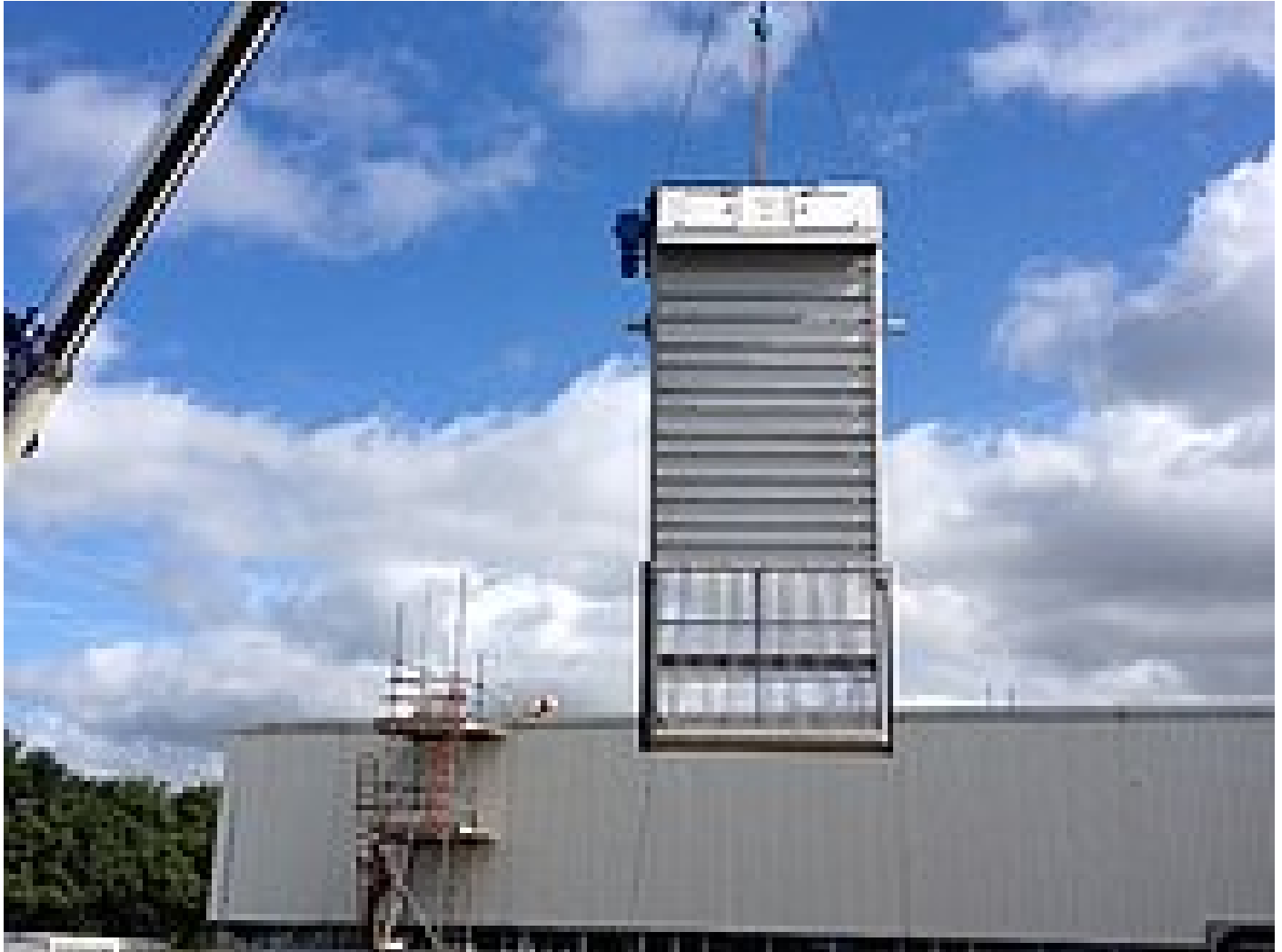
RakeMax® installation had to be completed through the roof of the building
