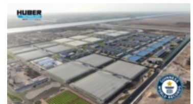
Aerial photo of the Bahr El-Baqar plant ; © Orascom Construction PLC and The Arab Contractors
