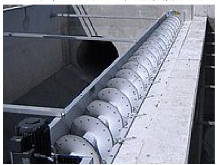
**Storm screens** are provided to retain solids at combined sewer overflows and reduce surface water pollution. Their power consumption is very low since they operate only periodically (See HUBER Storm Screens).
