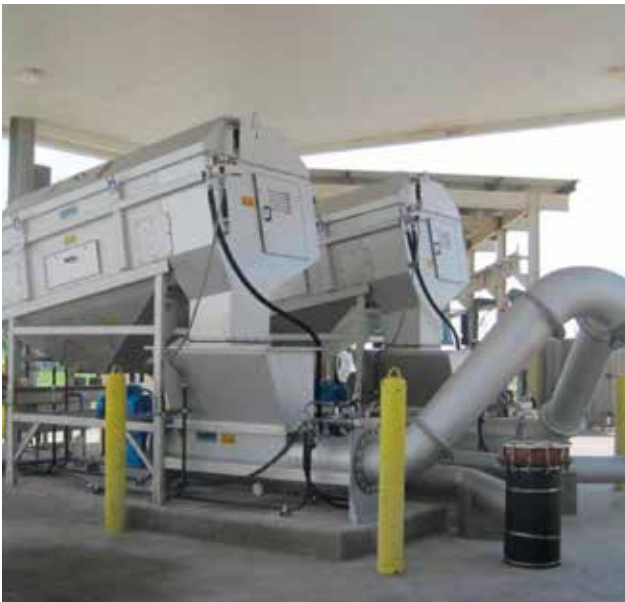
HUBER Wash Drum for washout and separation of all coarse material > 10 mm.
