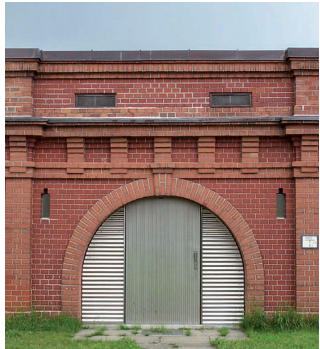
Attack-proof door type TT2.1, with segmental arch and side infills
