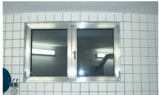
Double tilt window F 3, designed to prevent thermal conduction
