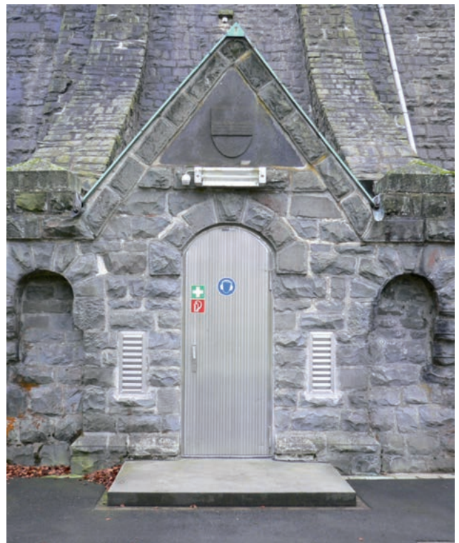
Attack-proof door type TT2.1, arch door, rigid louvres type TT10
