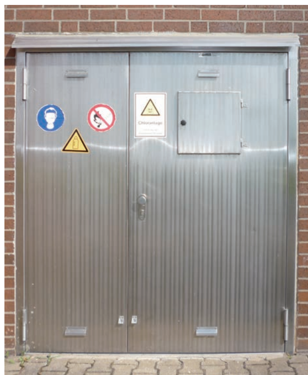
Chlorine room door type TT5.2, with covered window
