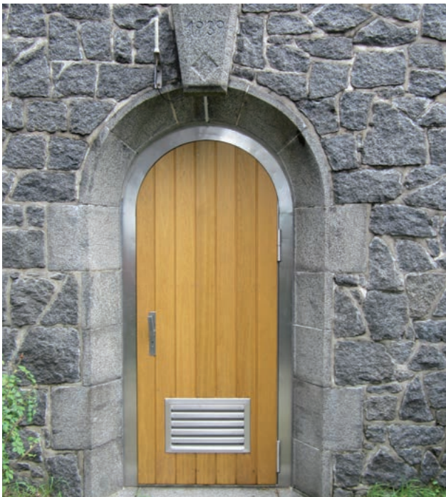
Attack-proof door type TT2.1, arched door with wood panelling
