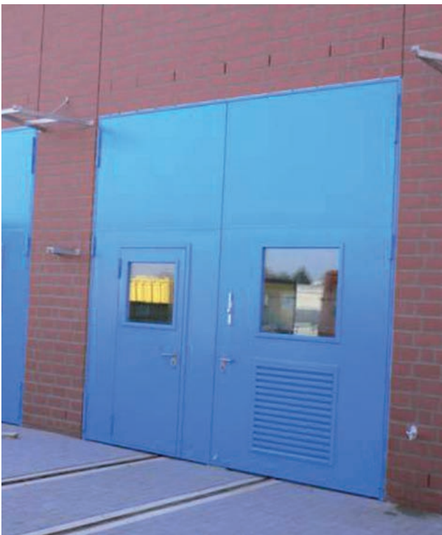
Exterior door type TT1.2, double-leaved, with louvre and wicket door, painted
