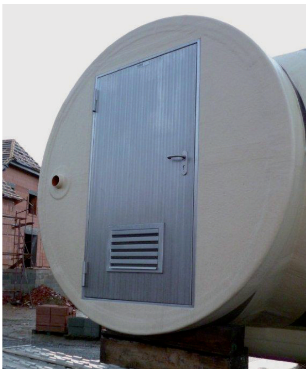
Exterior door type TT1.1, with louvre, installed in a GRP tank
