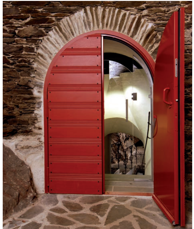
Attack-proof door type TT2.2, arched door with wood panelling, painted
