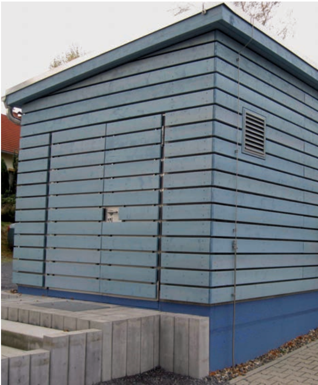
Exterior door type TT1.2, integrated in a wooden facade
