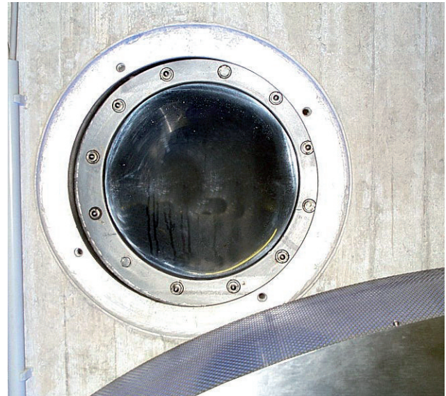
Inspection window type TT8, inside diameter 400 mm
