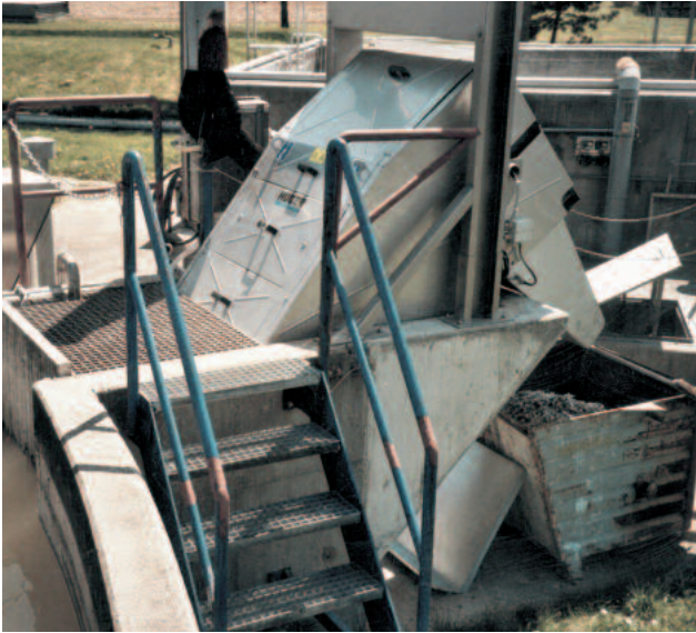
MD Paper Factory, Germany: solids / suspended material separation with HUBER STEP SCREEN® SSF
