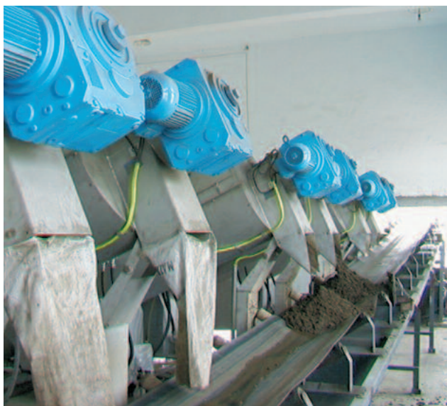
Paper factory Lingaong, China: dewatering of primary / biological sludge to > 28 % DS with HUBER ROTAMAT® Sludge Dewatering Plant RoS 3
