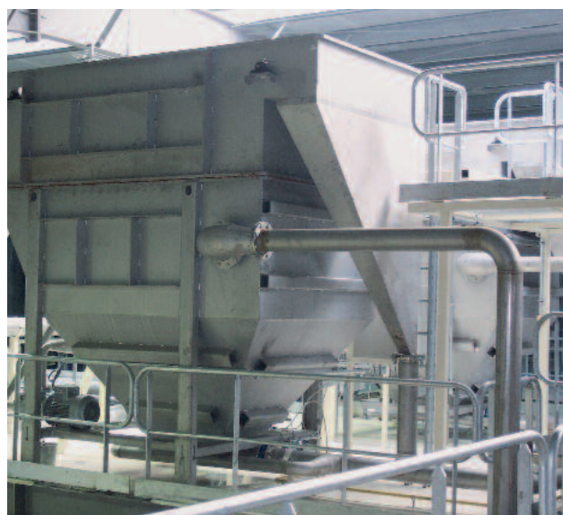
Paper factory Kronostar, Russia Dissolved Air Flotation Plant HDF-7 throughput: 70 m 3 /h
