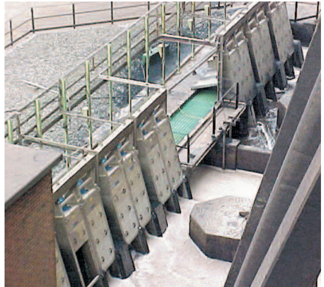
River water extraction in front of cooling towers with HUBER STEP SCREEN® SSV, Sasol South Africa
