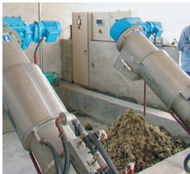
Paper factory Lingaong, China: mechanical preliminary treatment with HUBER ROTAMAT® Rotary Drum Fine Screen Ro 2, 1 mm, solids retention > 60 %
